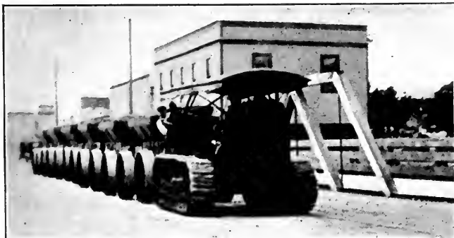
HAULING GRAVEL TO HIGHWAY JOB
